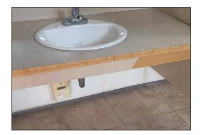
The restrooms did not smell fresh and clean and some of the laminate and fixtures need repair.
